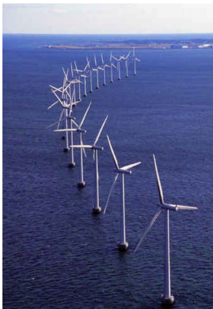
Figure.3.9.- Middelgrunden wind farm (2 MW, 20 wind turbines), Copenhagen, Denmark.
